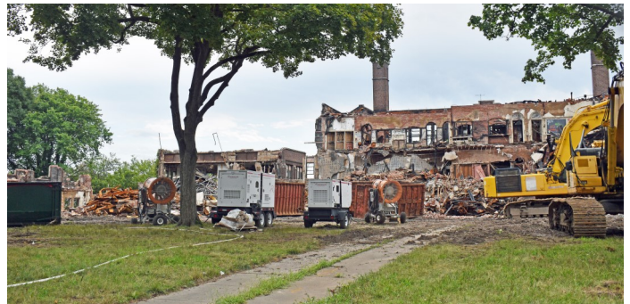
Demolition August 2024—Photo by Karl J. Flesch
